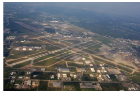
7800 Airport Blvd · Houston, TX 77061 713.640.3000 Fly2Houston.com/HOU
